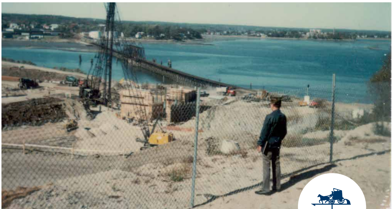
Construction of the East End Wastewater Treatment Facility which opened in 1979.
