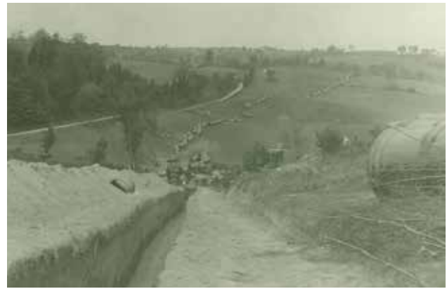
New Water Transmission Main being constructed in 1912
